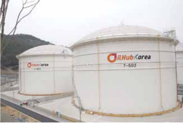
OKYC storage facilities OKYC 的储罐设施
