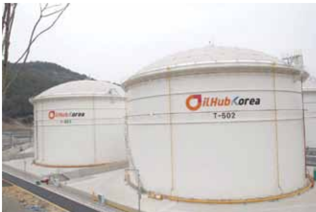
OKYC storage facilities OKYC 的储罐设施
